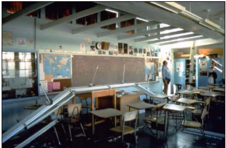
Damage to non-structural components of a school in the Northridge earthquake.
